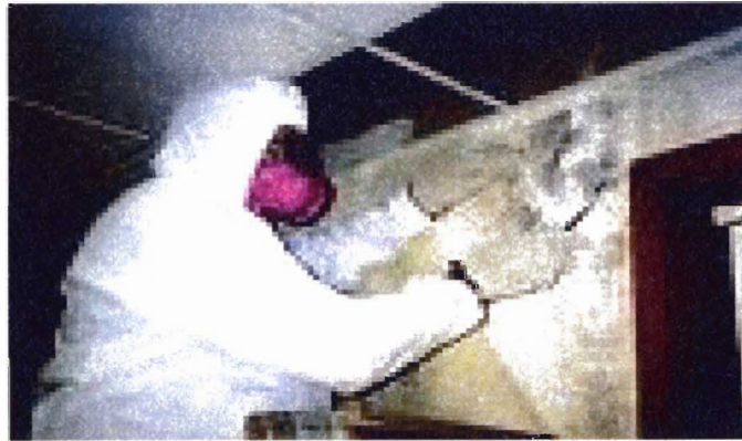
Figure 5. Photographs of a Mold Remediation Project
